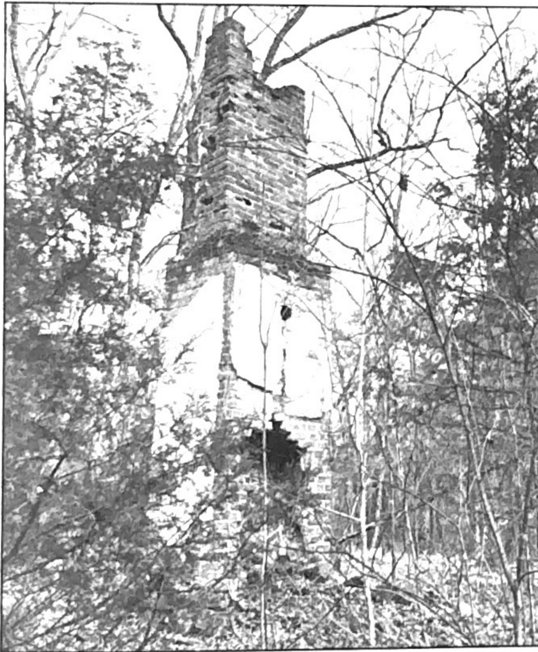
Chimney of the miller's house on Mill Creek in western Hanover; this site is on private property.
