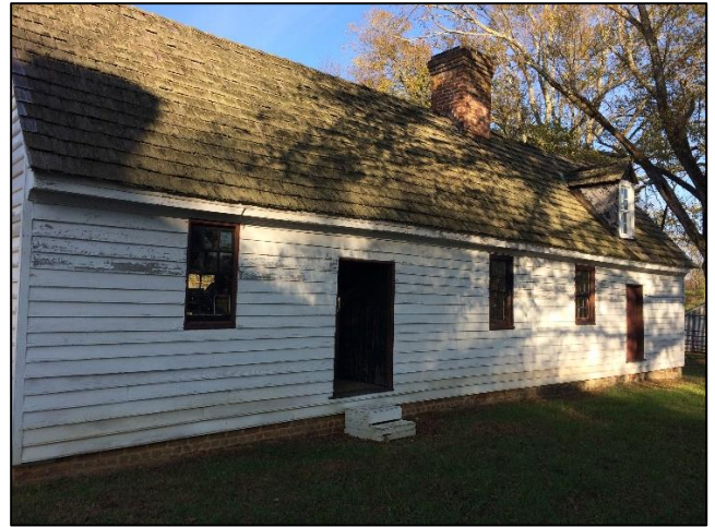
Pine Slash: ca. 1750 section at left; Addition, ca. 1800, with dormer at right
